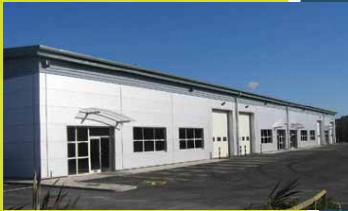
(Library photograph of Marrtree development at Glasshoughton Business Park, Castleford)
